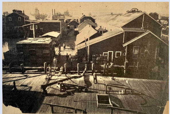
Original Booth Cannery with River Barge Docked in Foreground Building at the Extreme Left Later Replaced by a Concrete & Steel One Source: Fishing II Binder, Pittsburg HSA Library
