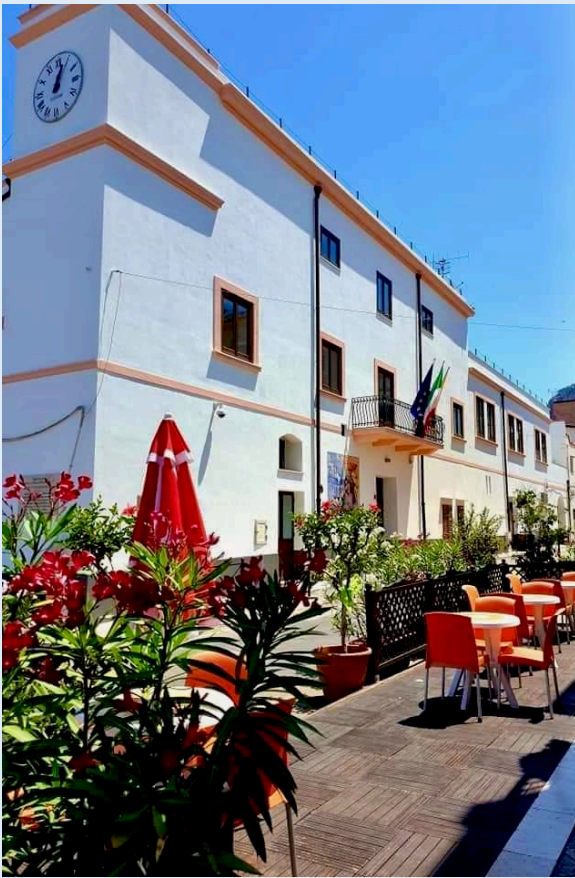
Isola's Completely Refurbished Palazzo Comunale, The Inland Face with the Entrance in View.
